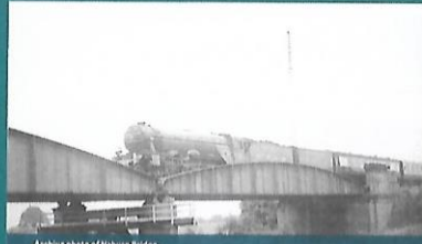
Archive photo of Naburn Bridge.
